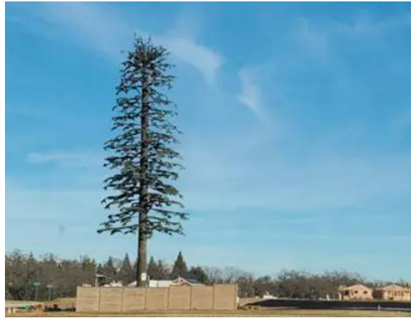
The kind of Monopine cell tower that will allegedly harm Los Osos residents.
